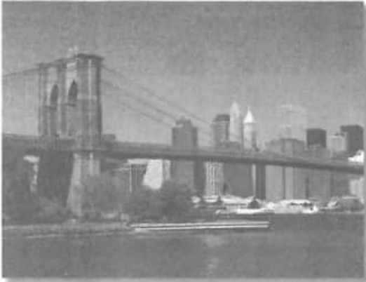
The Brooklyn Bridge, New York City
